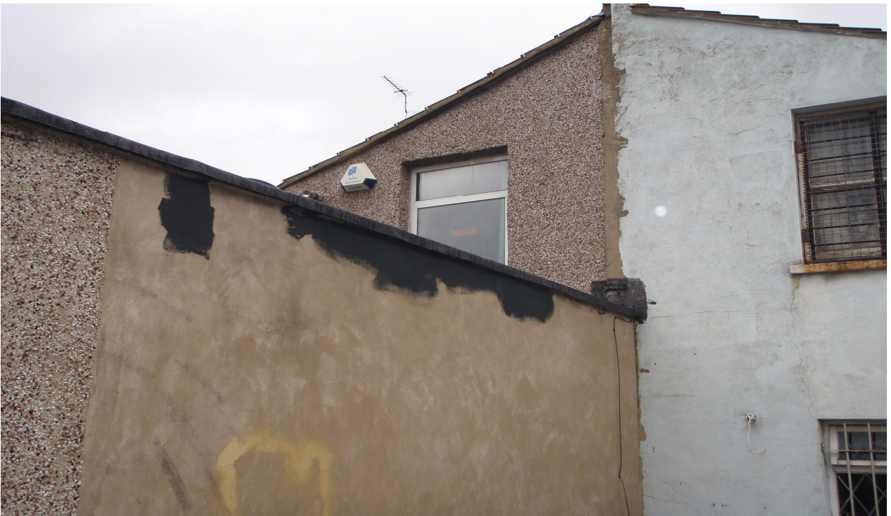
The flat roof area is the roof of the rear room area of the premises. The first floor is a commercial office property.
