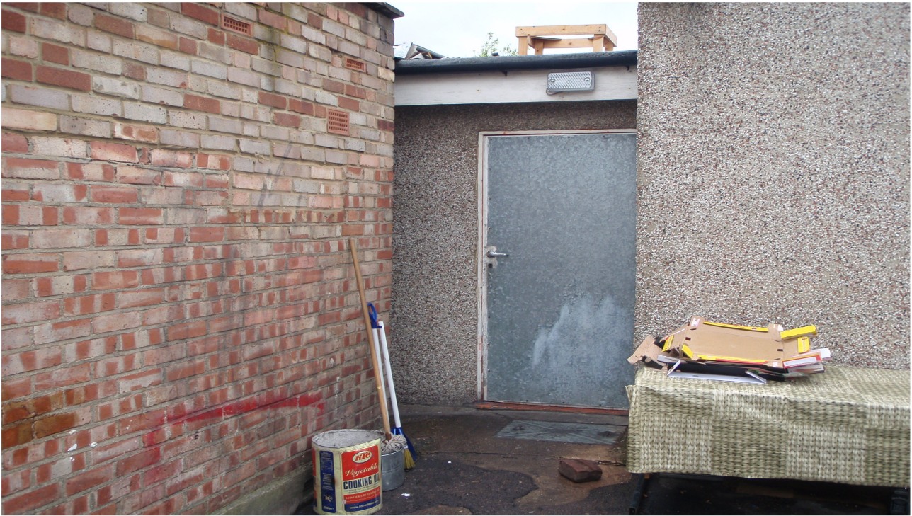
View from outside the rear emergency door.
