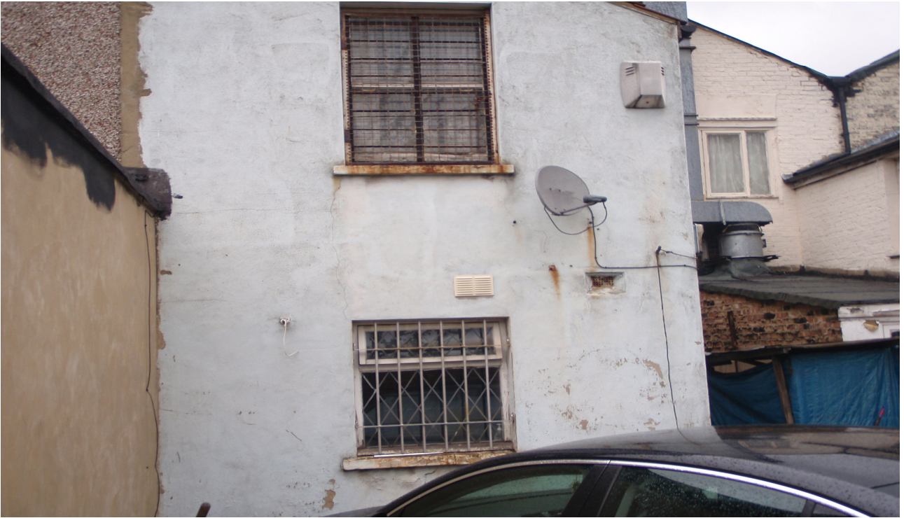
Rear of next door shop premises. It appears that the first floor is not residential.
